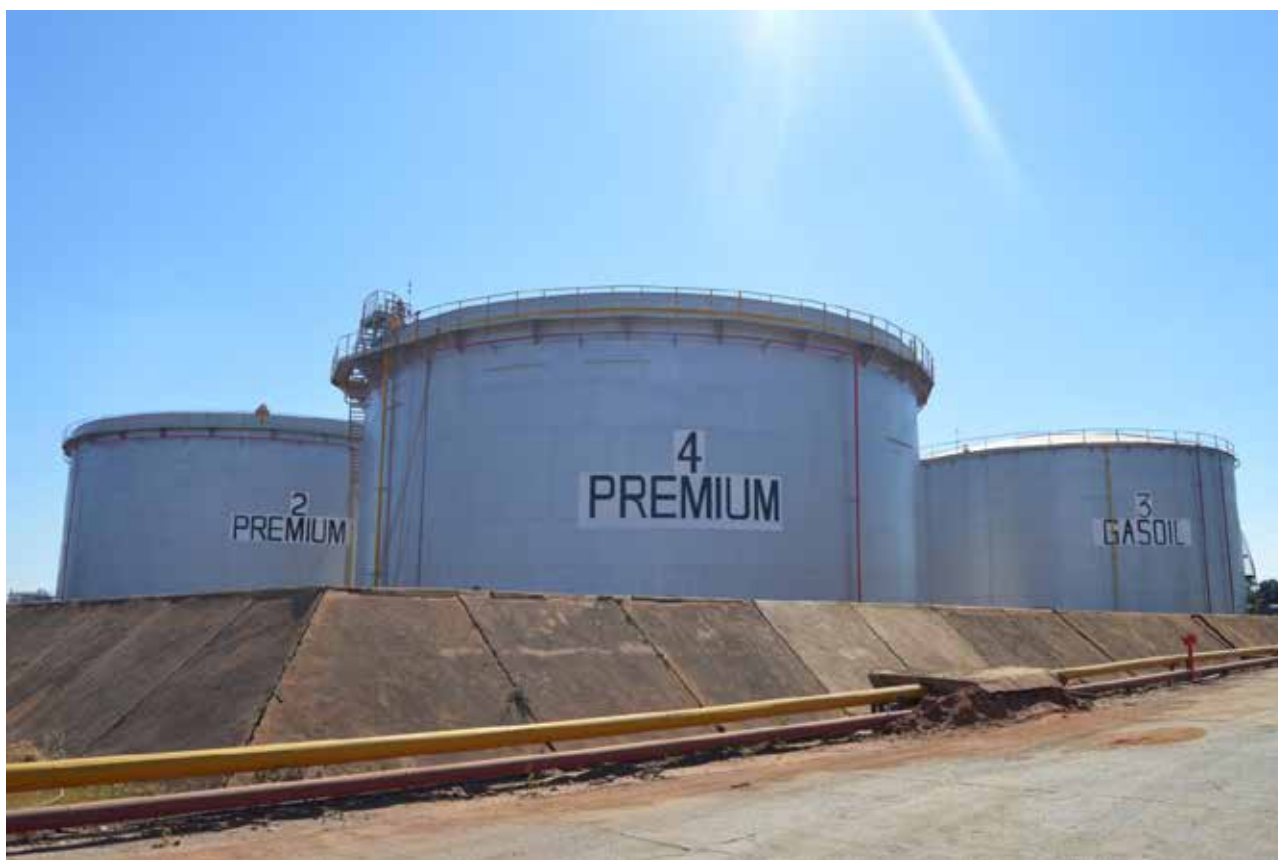
Petroleum products bulk storage
