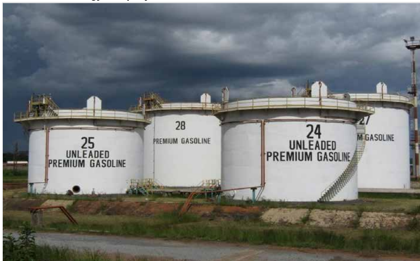
Storage tanks at Indeni
